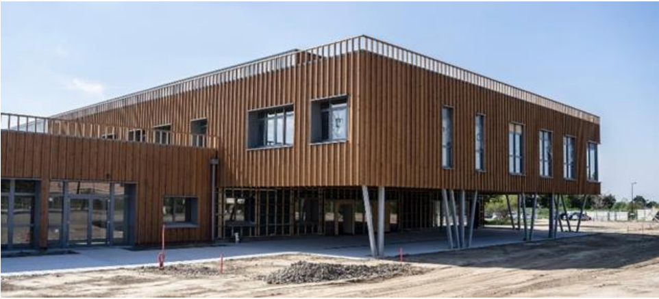
High school of Aizenay in Vendée (Pays de la Loire, France) built with wood and straw insulation - © Regional Council of the Pays de la Loire
